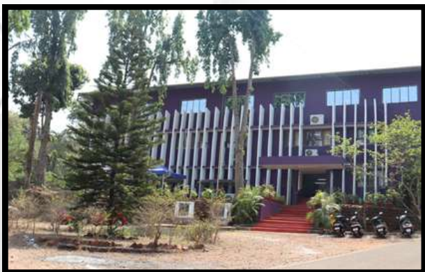
The Institute Building
