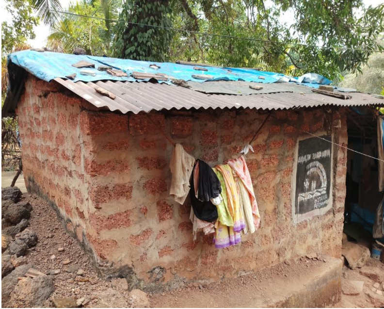
IAY house in Salcete Block
