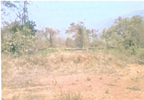
1 st Stage of cleaning and land development around Matoshri Anandibai Vaman Marathe Vidhyamandir School at Tamsado in V.P. Dharbandora.
