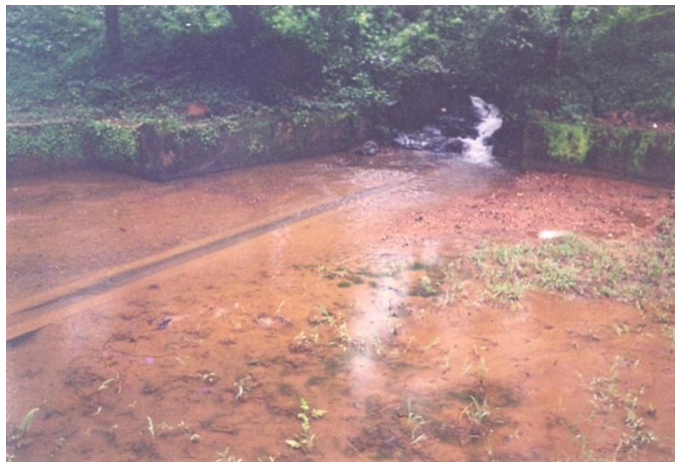
Clean and beautiful look of tirthachi tali after work done under MGNREGS.
