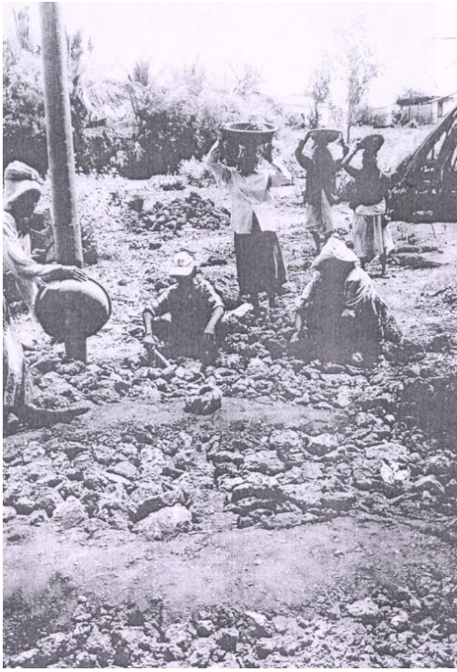
A group of women beneficiaries involved in repair of katcha road.
